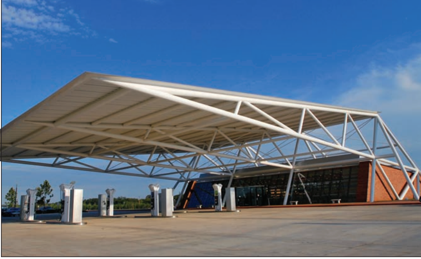
INTO INFINITY AND BEYOND: Part architectural statement, part practicality, a 110-foot steel cantilevered canopy juts over Pops 66 and its fuel island, pointing toward the future of the iconic Route 66.
